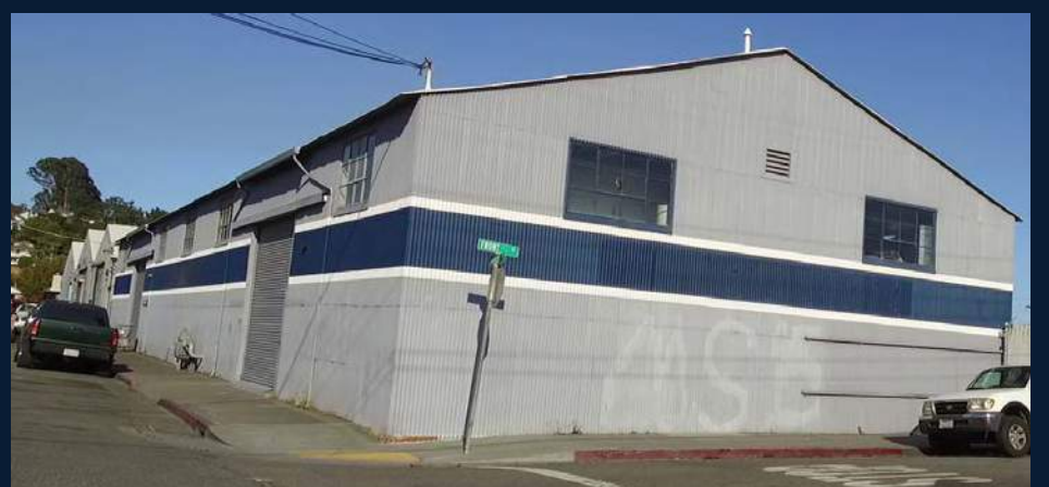
Industry and commercial businesses throughout low-lying area
