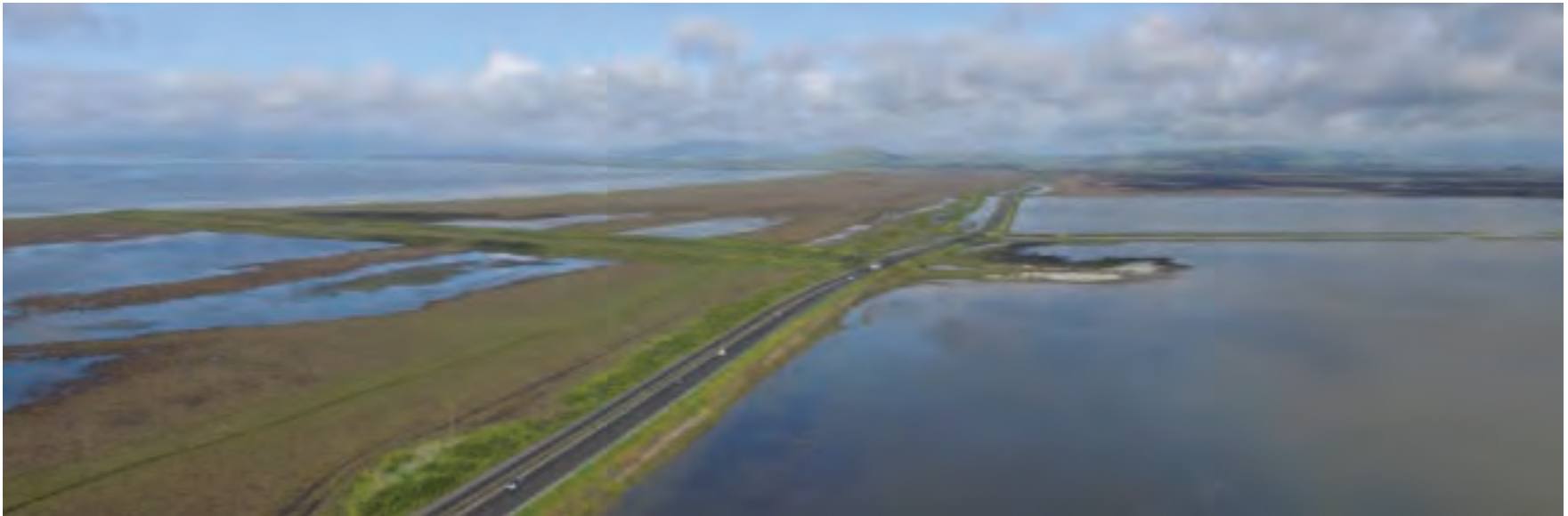
Low-lying SR 37 corridor as seen from Vallejo with the baylands on its right and San Pablo Bay on its left.
